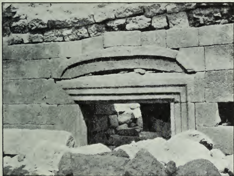
FIG. 17.—No. 3, door from narthex into nave.
